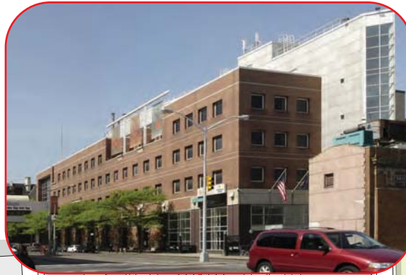
Building A: 475 Grand Concourse
